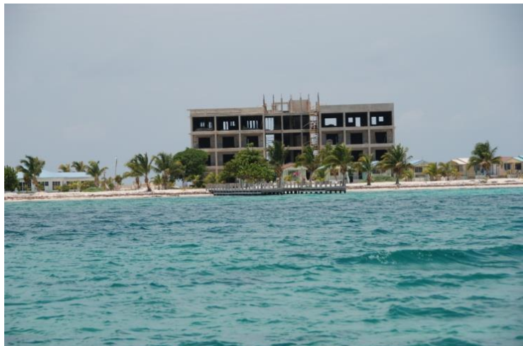
Sir Hakimi’s Belize Dive Haven (under construction)
